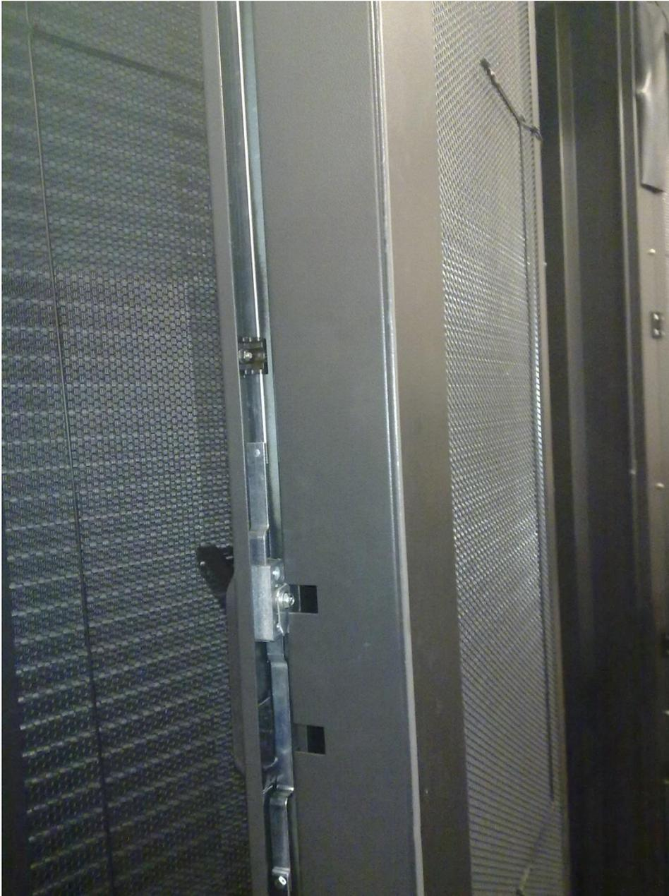
This shows the rear cooling panel of a cube rack. Note the thickness of the door.
